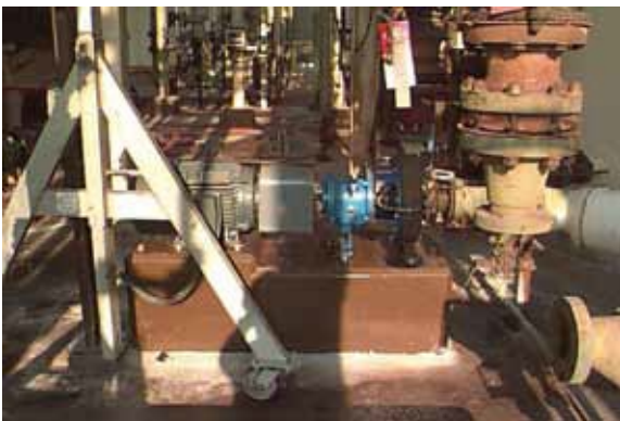
Figure 7. ANSI Chemical Pump on New Pre-Cast Baseplate/Foundation
