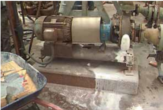
Figure 6. ANSI Chemical Pump on Flexible Base
