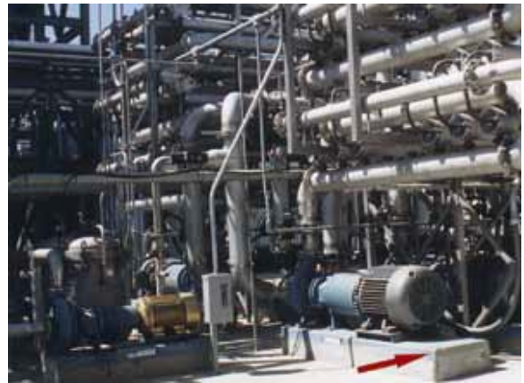
Figure 12. ANSI Pump – Channel Baseplate
