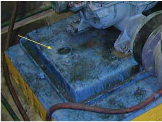
Figure 11. Grout Hole
